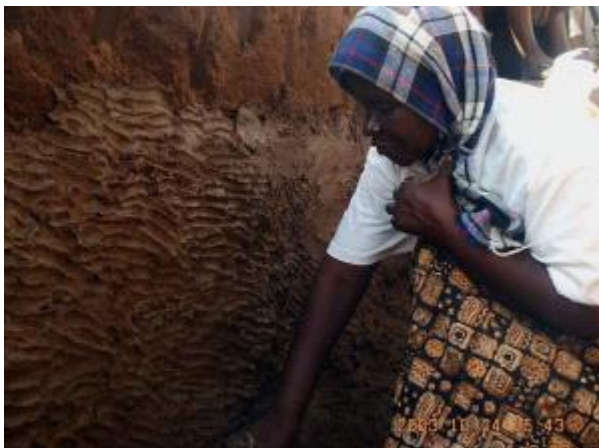
Picture 3: Tank lining/ Plastering ©Practical Action/Douglas Gumbo
